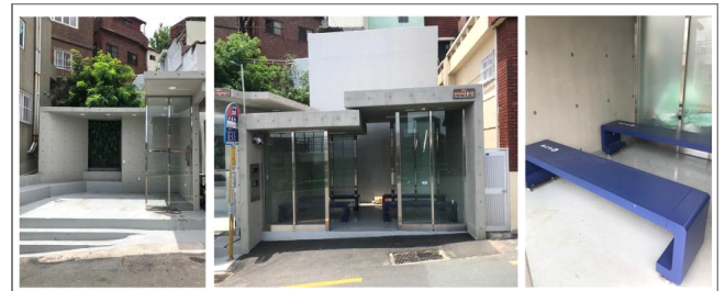
Figure 22: New Bus Stop (Community Space)
